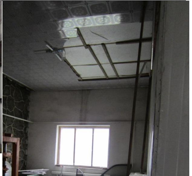
Pic 1.2 Ceiling with laminated sheet and Styrofoam sheets above
